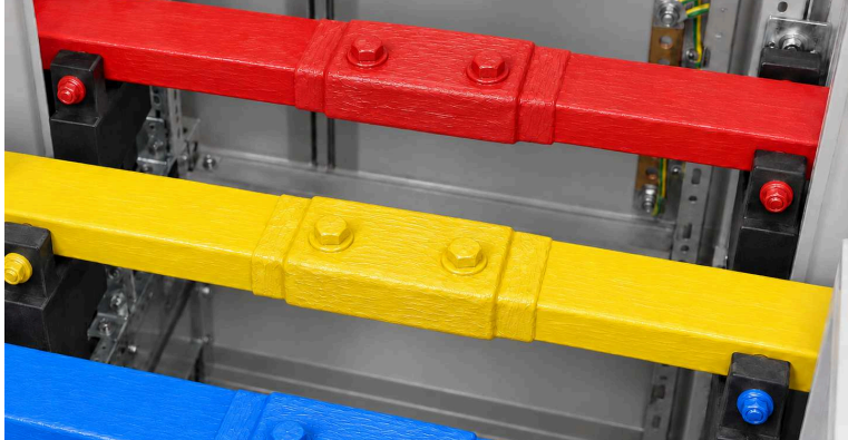
AFTER: JOINT & BOLT COATED
