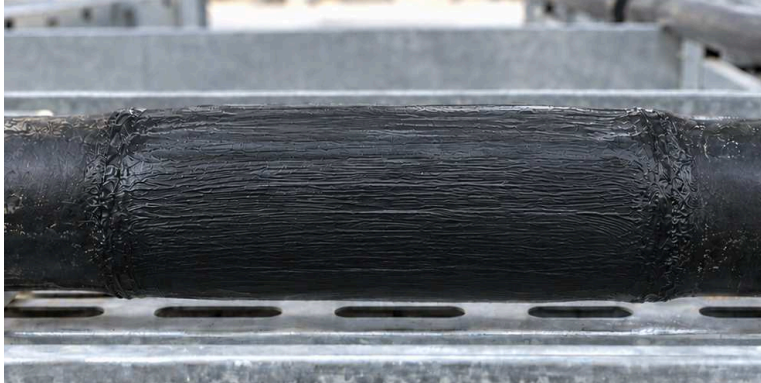
AFTER: LOCAL 931B REPAIR
