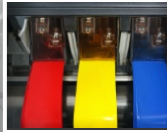
CLEANING, INSULATION AND PROTECTION
