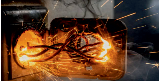
Where fire begins — a live electrical fault.
