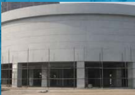
CONCRETE REPAIRS & PROTECTION
