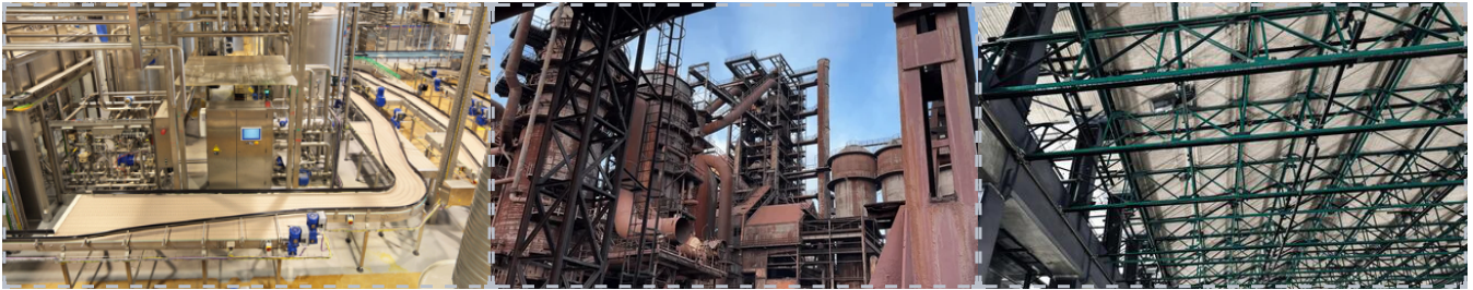
Steel above open product — grit can never fly Machines that never stop — and never get prepped Painting over inventory: prep impossible
