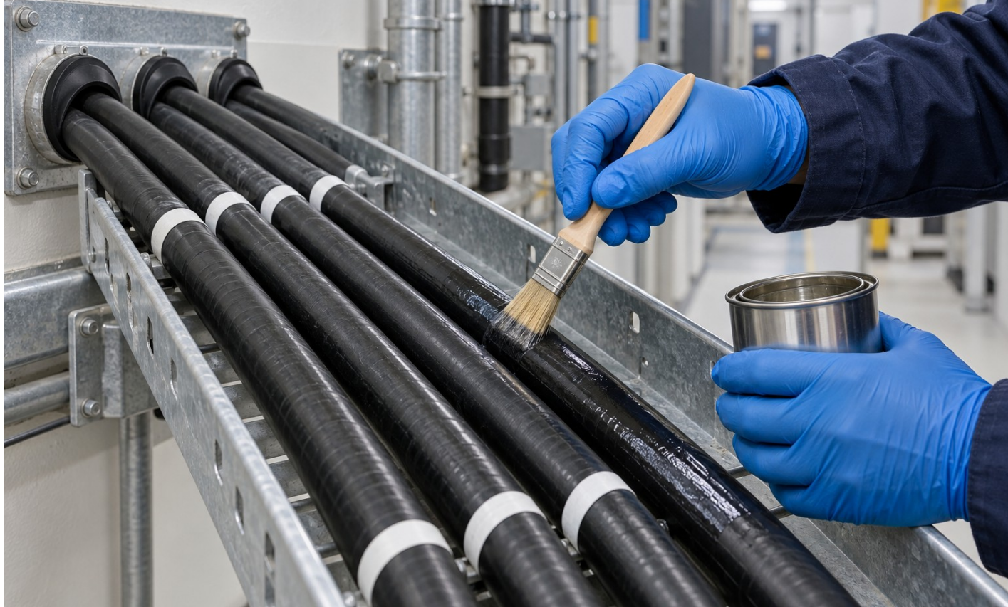
Coating fixed cable sheaths.
