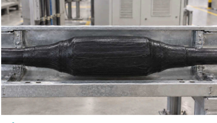
પછી: REPAIR & COATED
