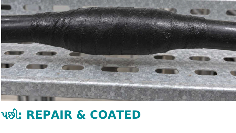
પછી: REPAIR & COATED
