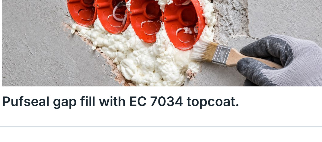
Pufseal gap fill with EC 7034 topcoat.
