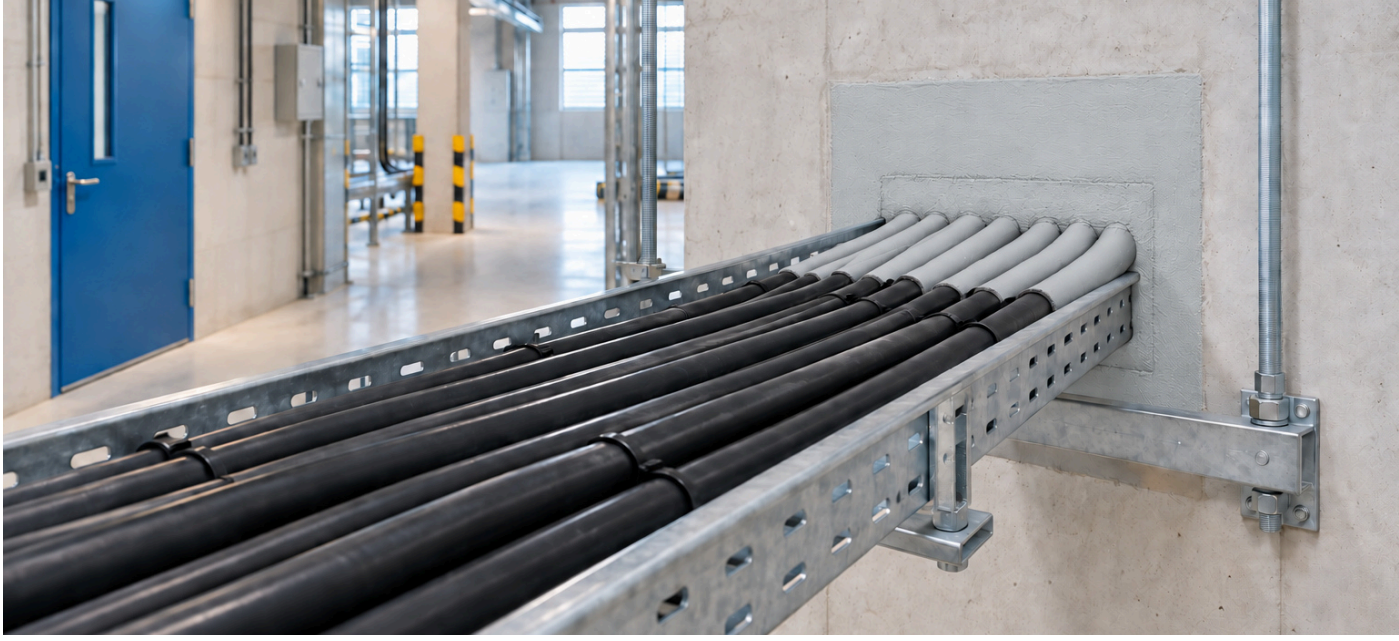
Sealed opening. Coated cables. Installation illustration.
