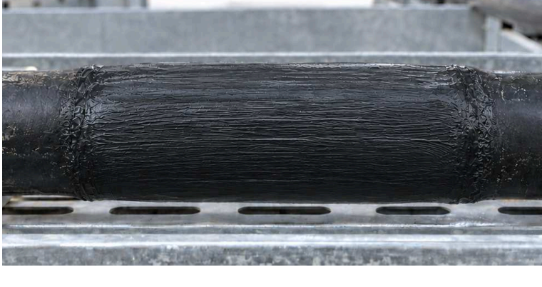
AFTER: 931B LOCAL REPAIR
