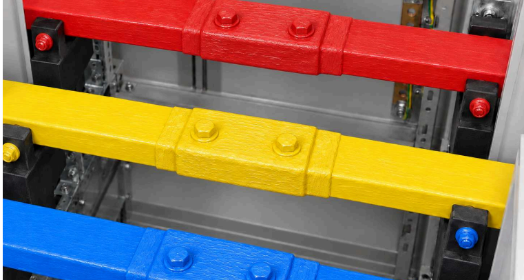
नंतर: COATED JOINT & BOLT
