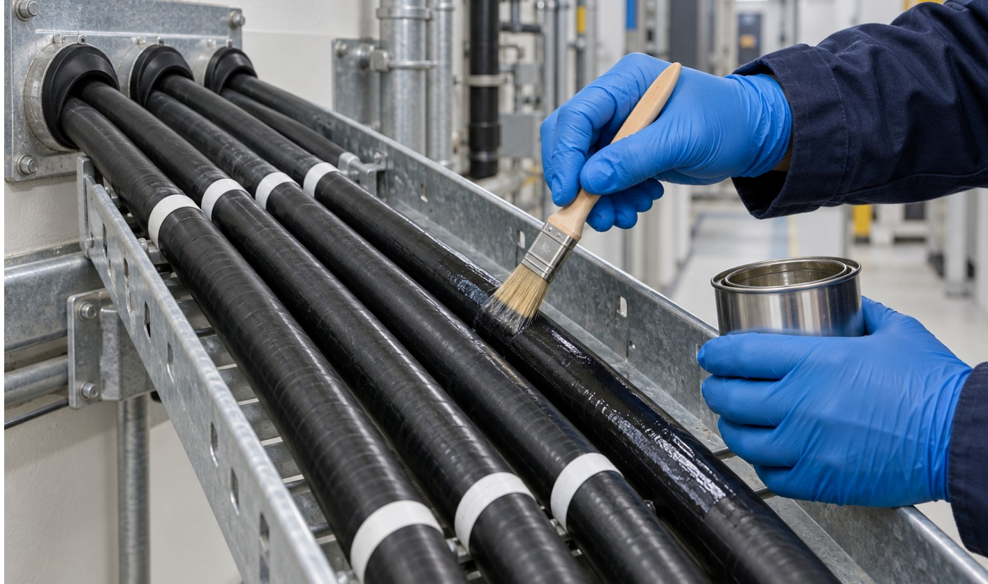
Coating fixed cable sheaths.
