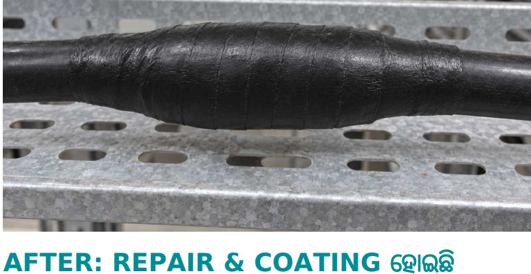
AFTER: REPAIR & COATING ହୋଇଛି
