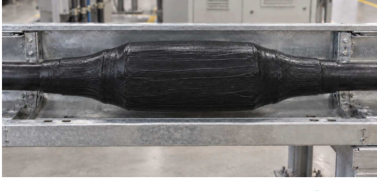
AFTER: REPAIR & COATING ହୋଇଛି
