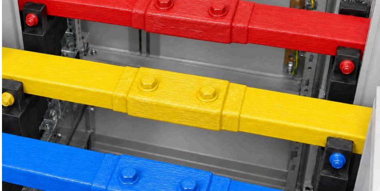
AFTER: JOINT & BOLT COATED
