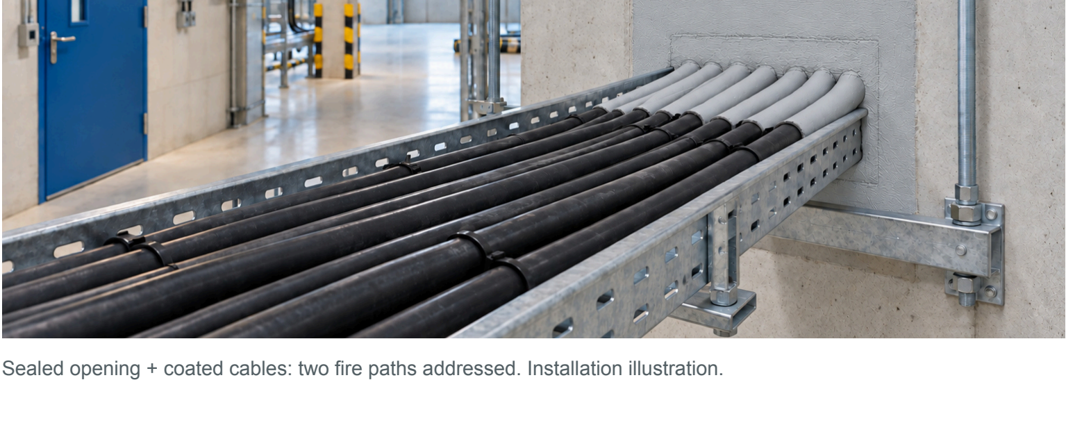
Sealed opening + coated cables: two fire paths addressed. Installation illustration.
