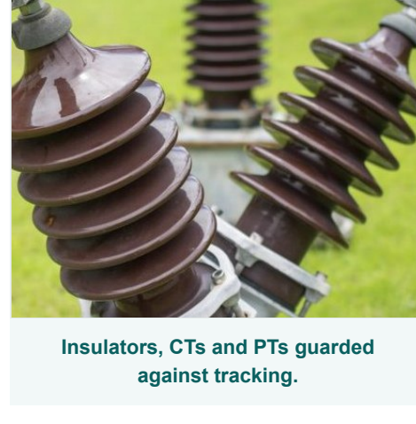
Deep-cleaning energised gear without flashover risk.
