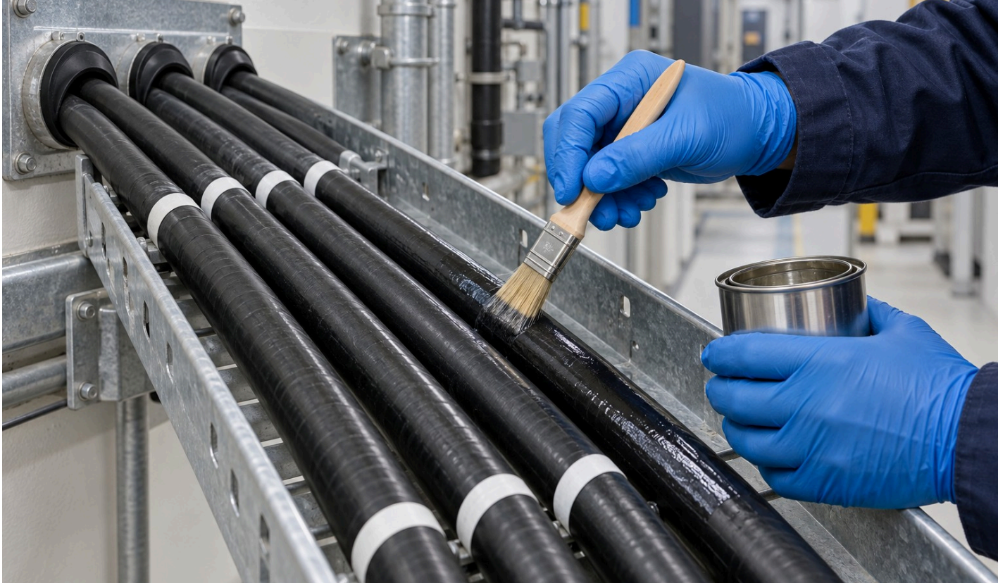
Fixed cable sheaths coating.
