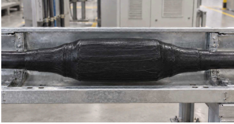
AFTER: REPAIRED & COATED
