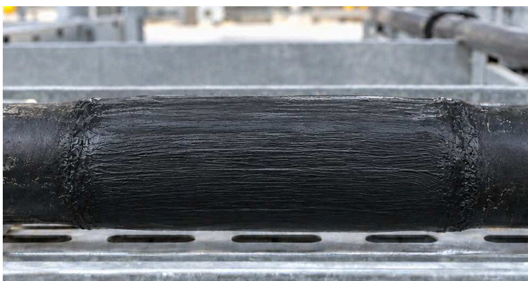
AFTER: LOCAL 931B REPAIR
