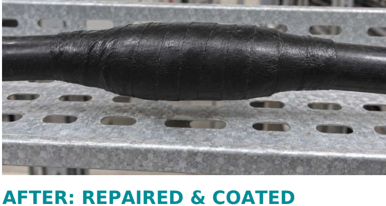
AFTER: REPAIRED & COATED
