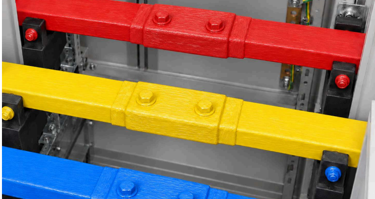
AFTER: COATED JOINT & BOLTS
