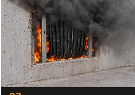
03 FIRE + SMOKE CROSS UNSEALED OPENINGS
