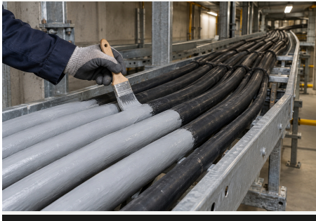
COAT CABLES. STOP FIRE SPREAD.
